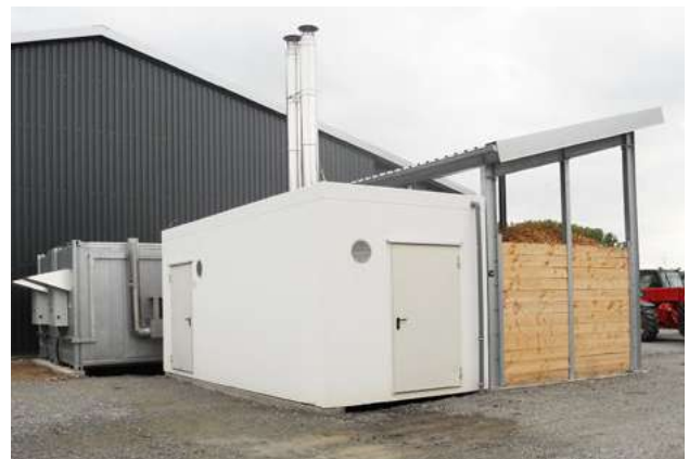
Single floor heating module 2 x 100 kW wood chips, business
