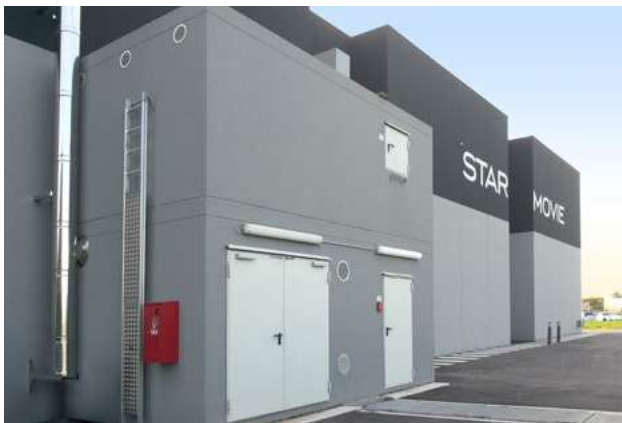
Double-floor heating module 200kW wood chips, business
